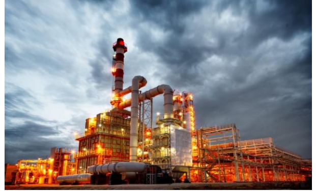
Oil & Gas Equipment
